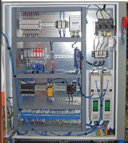
**I/O master distributors allow the use of a small control cabinet that only needs to house controllers, network switches, power supplies and safety relays. Photo courtesy Balluff Inc.**
